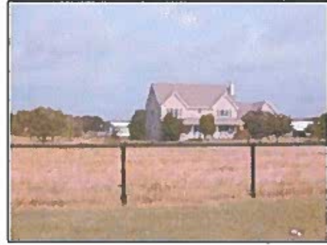
Example of Residential Estate Category
