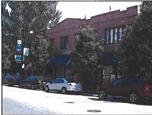
This attractive streetwall features parapets to shield rooftop HVAC equipment, on-street parking (with additional parking at rear), and sidewalk unbroken by driveways, large windows, awnings and street trees.
