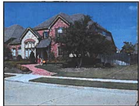
Home featuring a recessed garage not visible from the street. This home addresses all architectural concerns
