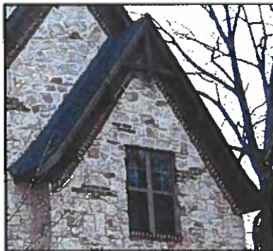
Steep roof pitch and a natural stone exterior address architectural guidelines
