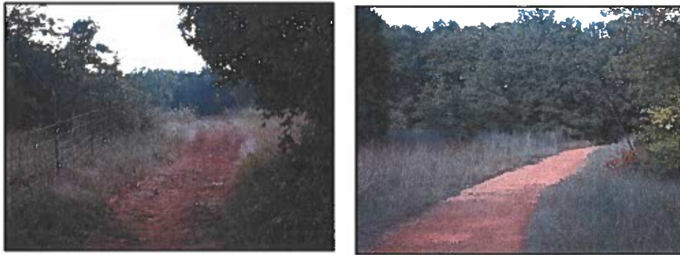
Common sections of trail. Widths along the existing trail vary from 6' to over 20' in some areas. Ensuring a minimum width of 10' gives continuous access to fire and EMS vehicles.
